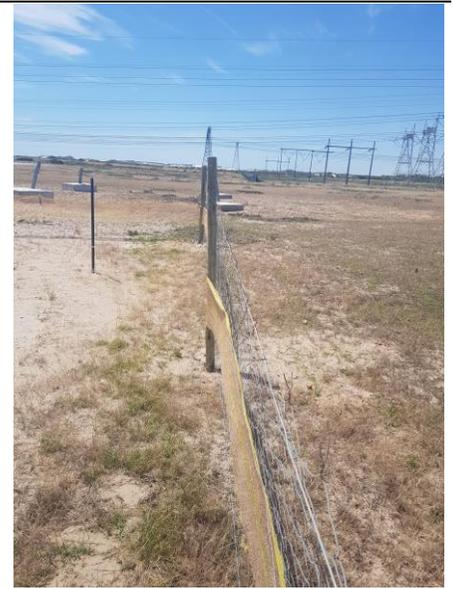
Image 12: Site barrier fence and cleanace of vegetation.
